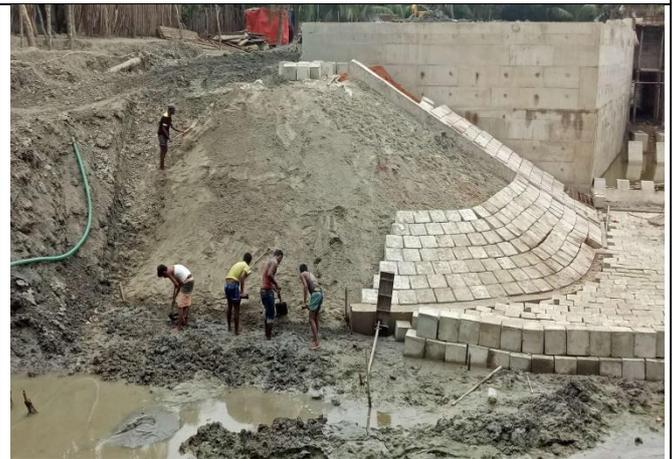
Figure 3-65: *Placing of CC block for DS-03 in Polder 40/2*
