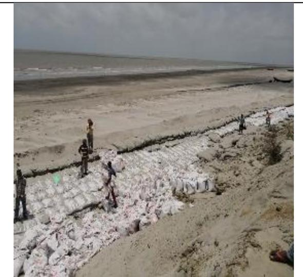
Figure 3-79: Synthetic bags placing for emergency slope protection work 31+280-31+408 in Polder 48
