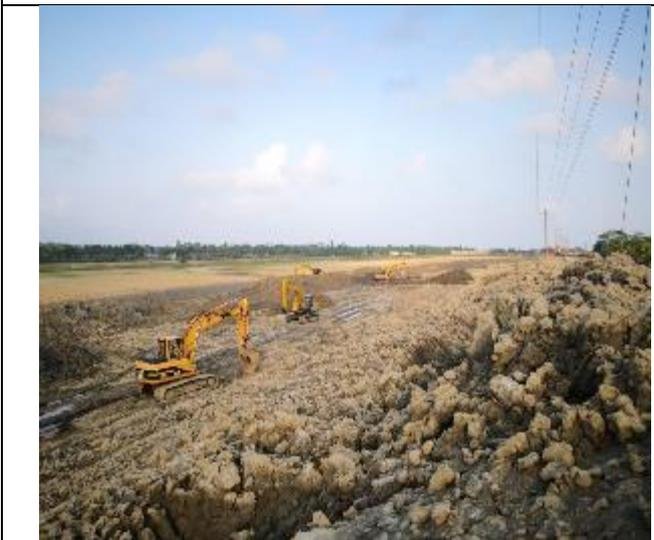
Figure 3-78: Earth work for embankment KM16+134-17+000 in Polder 48
