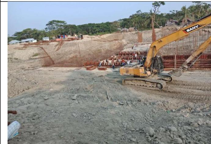
Figure 3-66: *Form work for end sill of DS-05 in Polder 40/2*
