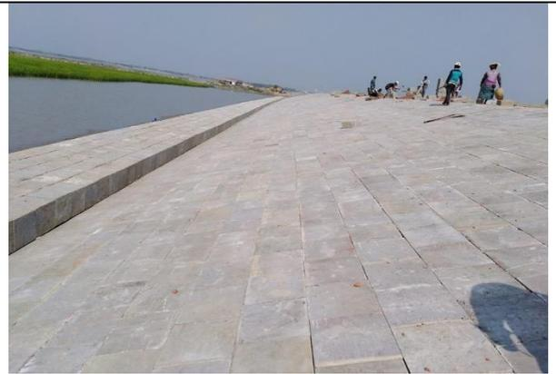
Figure 3-46: Completed Slope Protection Works in Polder-32
