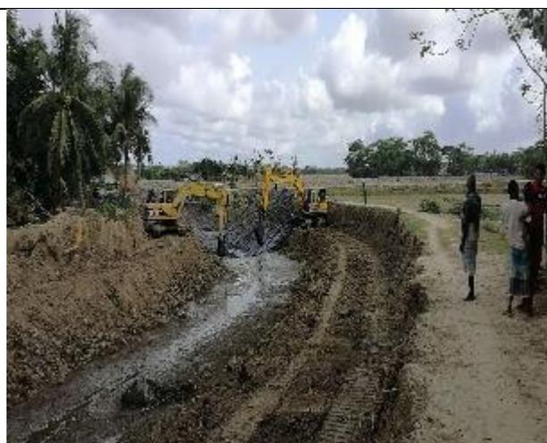
Figure 3-73: Excavation / Re-sectioning for drainage channel of DS-03 in Polder 47/2
